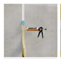
Fill the empty space with mineral wool and apply a layer of PIROSILICON 240 on both sides of wall
