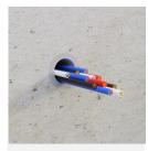
Run the cables inside the duct (the duct may be no greater than 60 percent of its cross section filled with cables)
