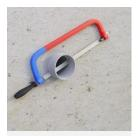
Cut off the parts of the **Piro Multitube EPipe** duct on both sides of the partition by means of saw
