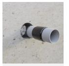
Place **Piro Multitube EPipe** in the hole so that its black part is centrally located inside the partition
