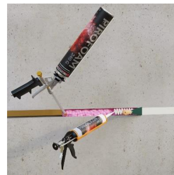
Fill the empty space PIROFOAM 240 and apply a layer of PIROSILICON 240 on both sides of wall
