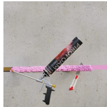
Fill the empty space with PIROFOAM 240 and cut the leftover material on the wall surface
