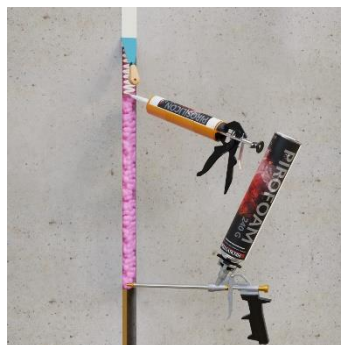
Fill the empty space with PIROFOAM 240 and apply a layer of PIROSILICON 240 on both sides of wall
