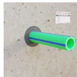
Mark the penetration with the attached label, mark the fireproof paste **PiroCoat I** on it, enter the date and name
