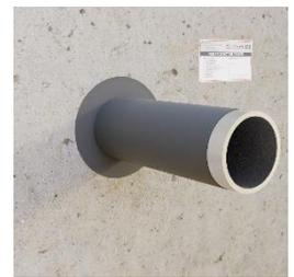
Mark the penetration with the attached label, mark the fireproof paste **PiroCoat I** on it, enter the date and name
