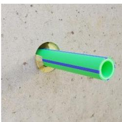
Fill the space between the pipe and the partition with mineral wool with a minimum density of 50 kg/m<sup>3</sup>, leaving 5 mm space from the front of the partition
