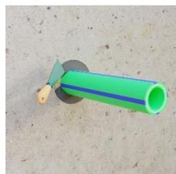
Apply **PiroCoat I** on the wool with a spatula and create a ring around the pipe, for wall thickness of min. 4 mm, for floor min. 5 mm and a width of min. 15 mm
