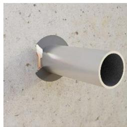
Using a brush, apply **PiroCoat I** on the partition in such a way that a ring with a width of min. 50 mm and a minimum thickness of 0.6 mm is created
