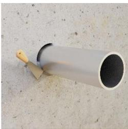
Fill the space between the pipe and the partition tightly. Use mineral wool with a density of min. 50 kg/m<sup>3</sup> or cement mortar
