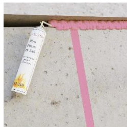
Fill the horizontal expansion joint tightly with Piro Foam PF 240
